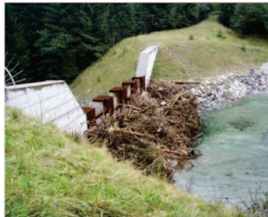
Figure 1: The problem of driftwood in mountain basin affected also by debris flows
