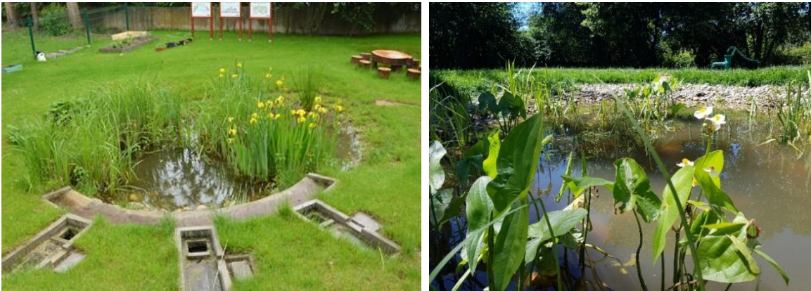
Picture 1, 2. Climapond in the Public Kindergarten No 16 in the city of Radom, Poland (construction: FPP Enviro, Poland within an EU project LIFE-RADOMKLIMA-PL, LIFE14CCA/PL/000101; property rights: P.419910, 20/12/2016).
