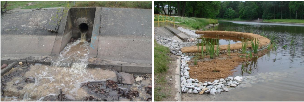
Figure 4. Hybrid system (separators and SSSB) purifying stormwater from at the outflow of stormwater sewage from a small sealed catchment. Due to lack of adequate space on land, the engineered part of the hybrid system (separators) are located on land, while SSBS part of the system directly in the reservoir (“instream”). Before (on the left) and after construction (on the right). LIFE08ENV/PL/000517 Project EH-REK. © T. Jurczak.
