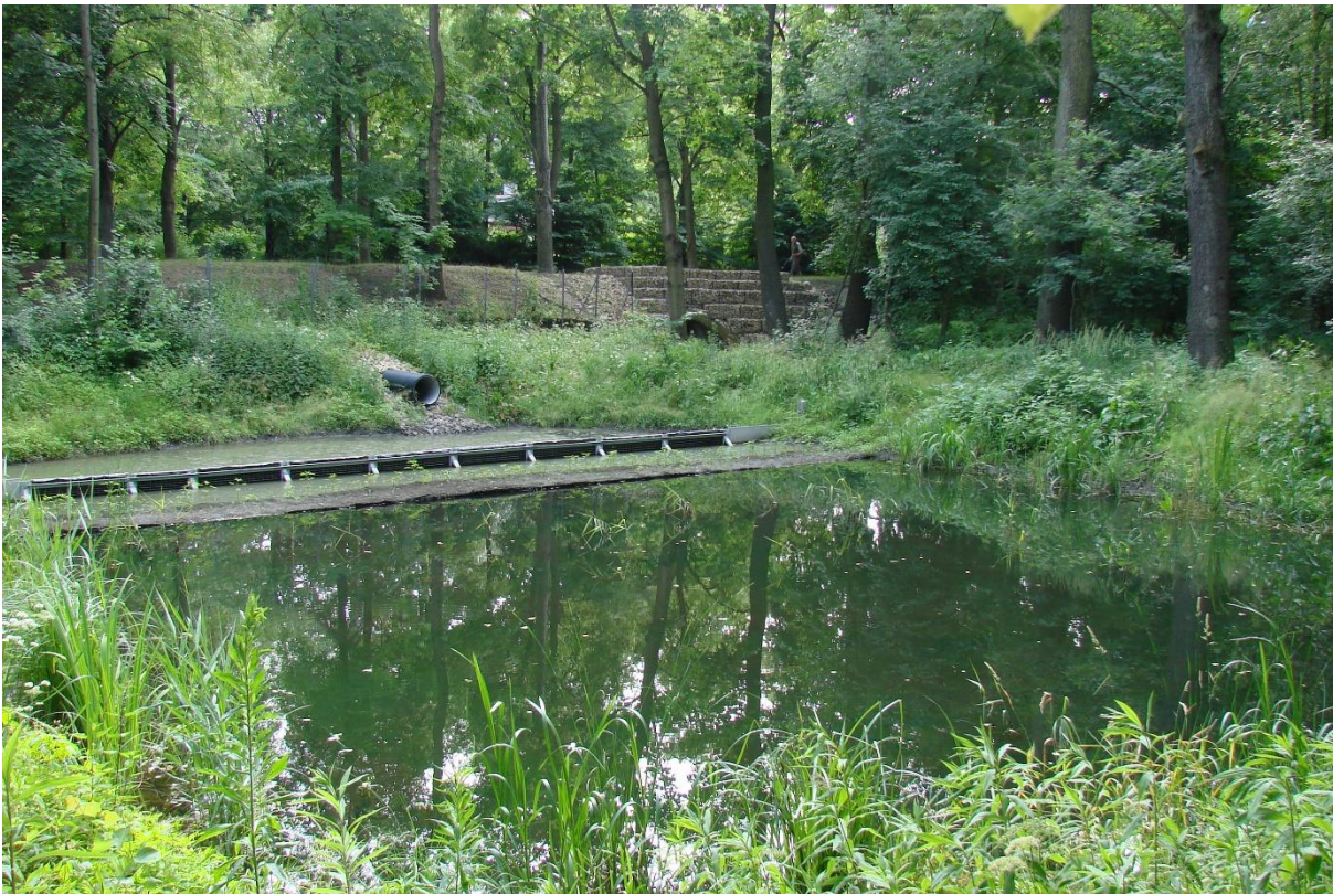
Figure 1. Sequential Sedimentation Biofiltration System, part of a hybrid system purifying stormwater runoff from a street in Lodz, Poland, before its disposal to recreational reservoirs at the Bzura River. SSSB implemented within LIFE08ENV/PL/000517 Project EH-REK „Ecohydrologic rehabilitation of recreational reservoirs ‘Arturowek’ (Łódź) as a model approach to rehabilitation of urban reservoirs”. © T. Jurczak.
