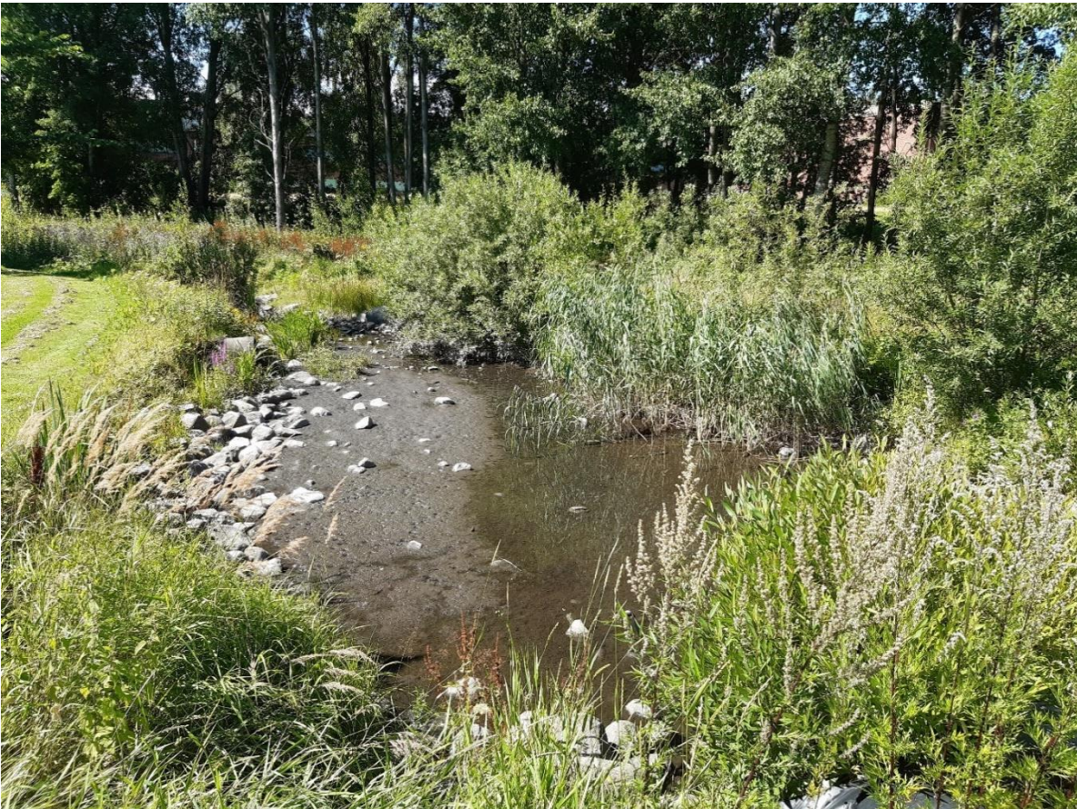
Figure 3. Water levels in the constructed ponds running to the main water system is low during summer, leading to appearance of bottom layer. © Jussi Torkko
