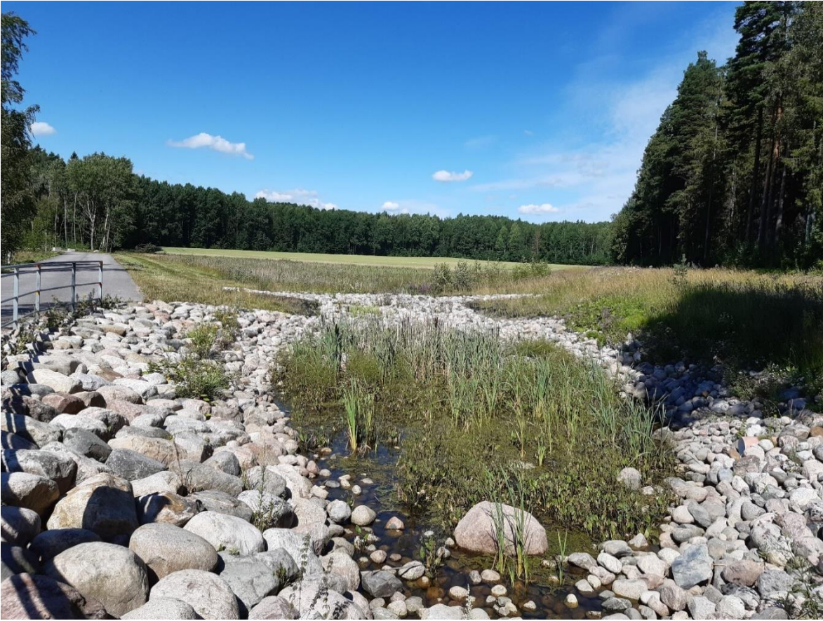
Figure 1. Murto stormwater basins. Smaller in the front and larger wetland area on the background. Stormwaters from Kivistö are directed here via a stream. In the future, the field on the background and surroundings is planned to provide housing for 2000 people which will increase the amount of stormwaters. The neighbourhood identity would be built around urban farming and sustainable stormwater control (City of Vantaa, 2020). ©Sonja Koivisto
