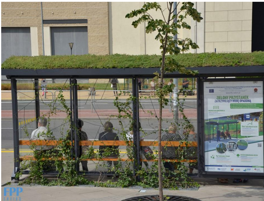
Picture 3. Green Bus-Stop with the excess of water directed to tree-tr trench in the city of Radom, Poland (developed and implemented by FPP Enviro, Poland).
