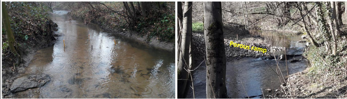
Figure 2.4. appearance of a porous ramp after construction. Left: sand accumulation upstream of the porous barrier; right: porous barrier, here made of pebbles.
