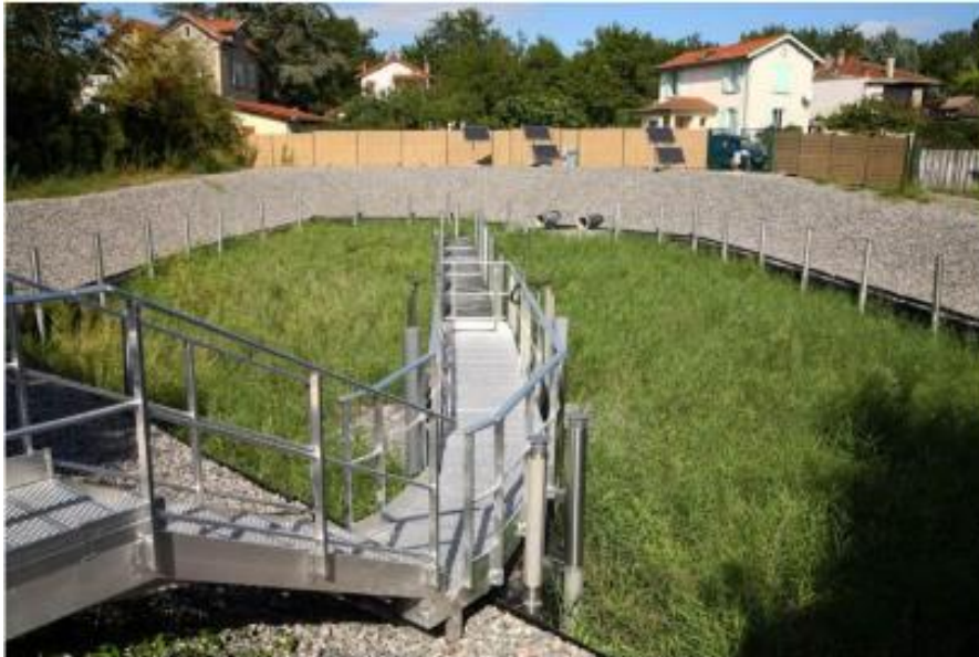
Figure 2.1. Biofilter to improve combined sewer overflows water quality, before rejection to small water courses 1 .
