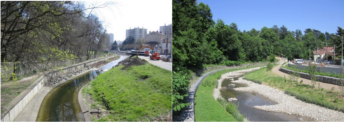
Figure 2.5 Before and after restoration of concreted watercourse in an urban area
