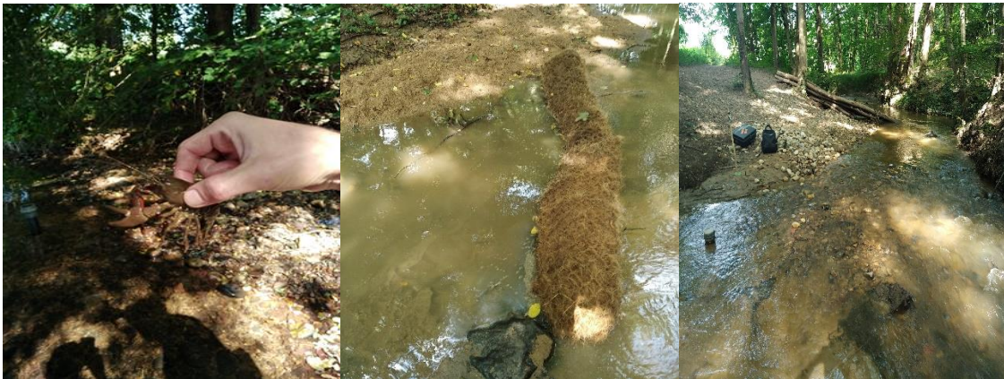
Figure 18. Local biodiversity to protect: crayfish (left). Coconut fiber barrier during the earthwork phase to limit water turbidity that can harm downstream aquatic species (center). Intrusive tree trunk device made by fishermen that helps destroy the porous ramp (right).
